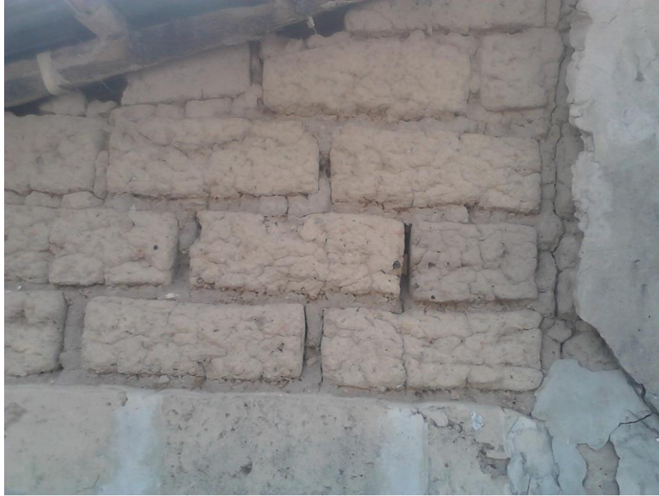
Figure 2.14: Typical Gambian Earthen Wall. The photo above illustrates the erosion of poorly made earth blocks when exposed to the Gambian wet season, Source (Author).
