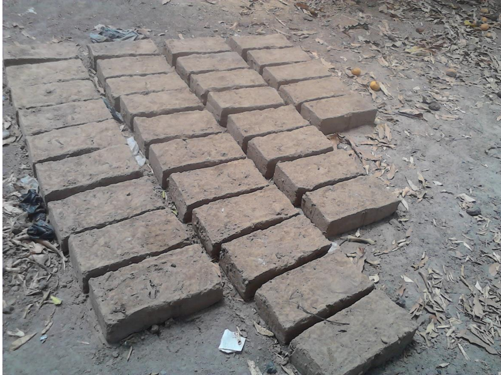
Figure 2.13: Gambian Earth Blocks: Newly cast earth blocks curing in open air in a construction site in The Gambia
